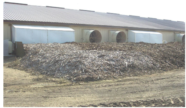
A biofilter, shown above, uses living matter to capture and biologically degrade pollutants expelled livestock production buildings. Photo by Rick Stowell, University of Nebraska/Flickr, CC License 2.0.
