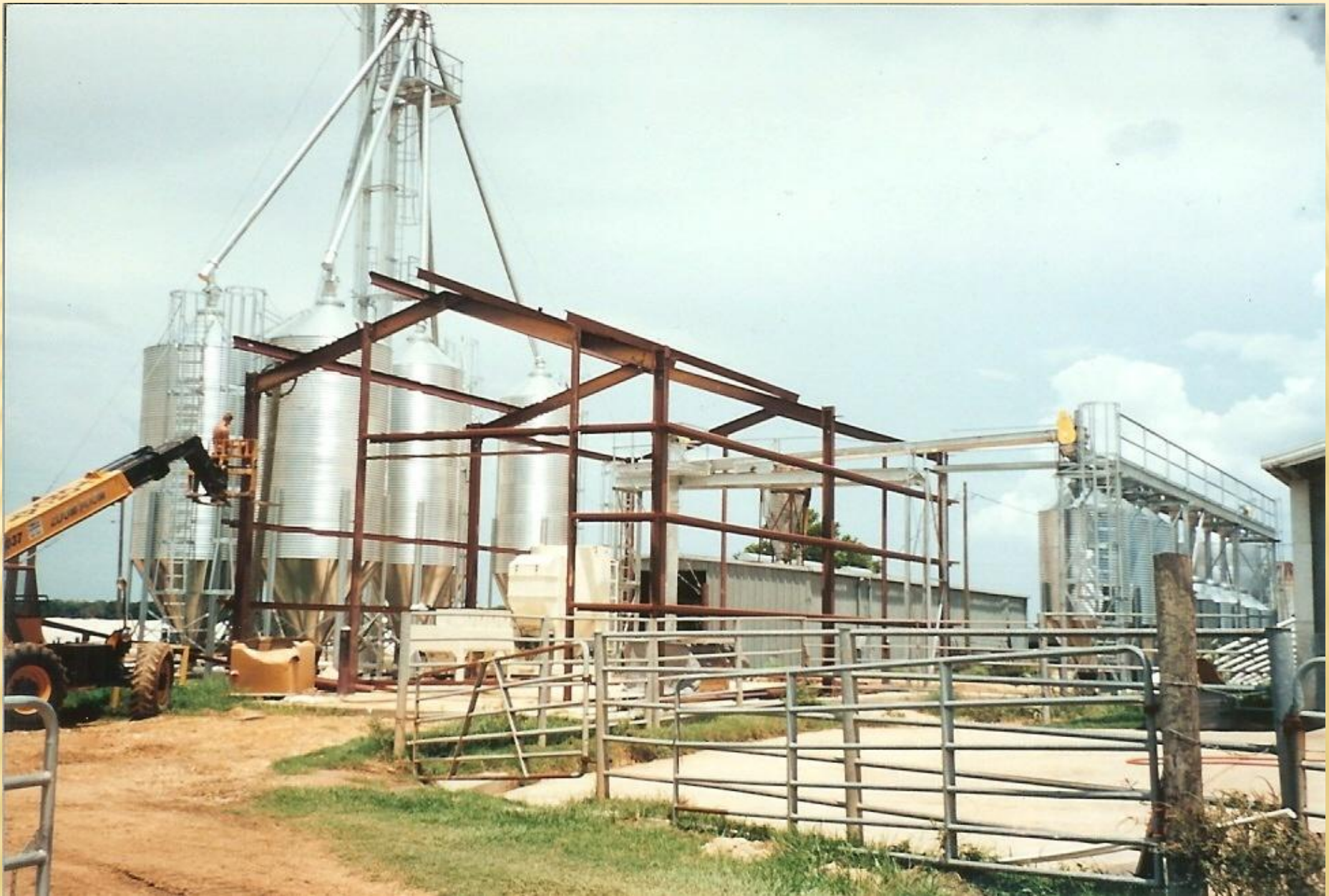
Feed Mill Under Construction – Franklinton, LA
