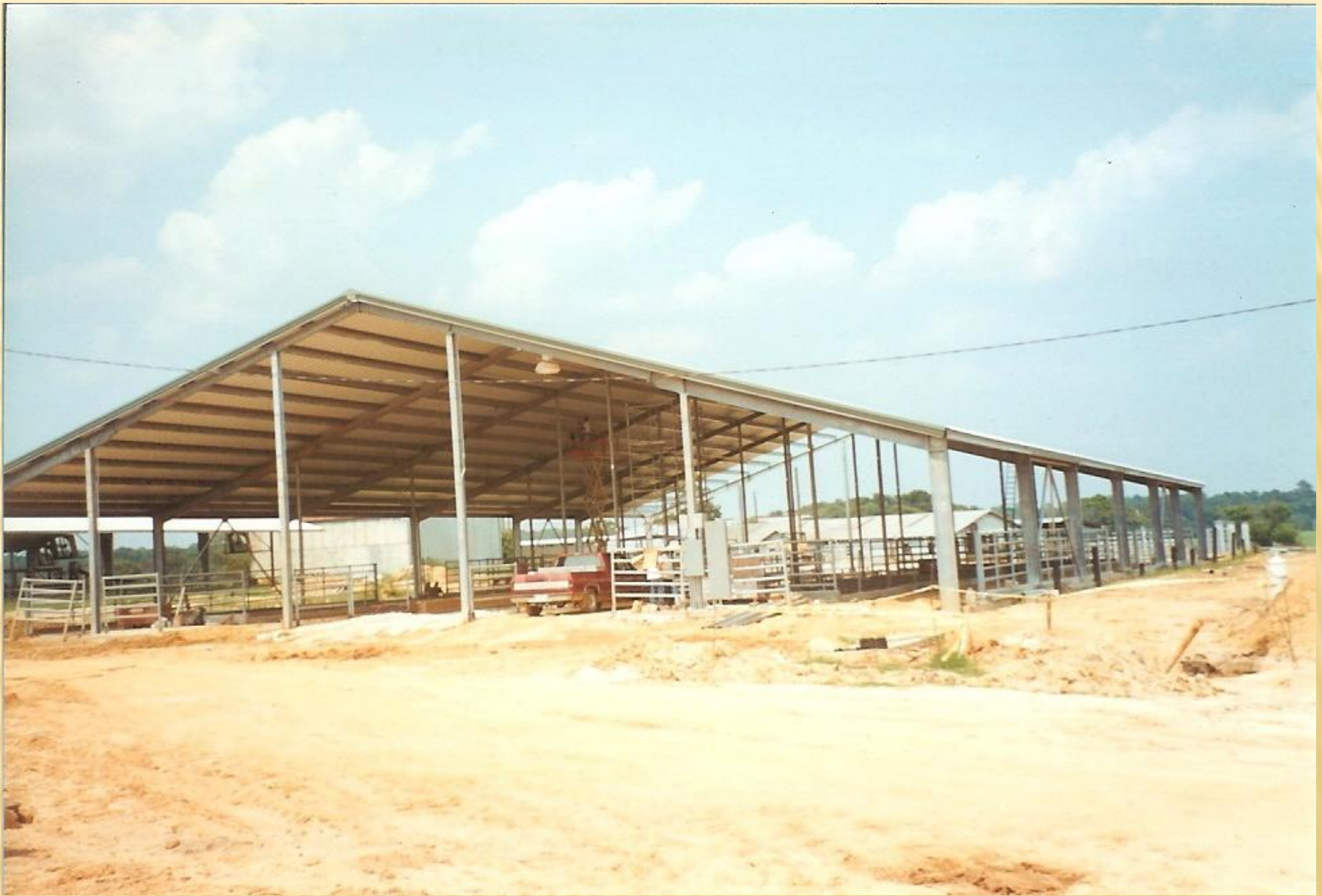
Freestall Barn Under Construction Franklinton, LA
