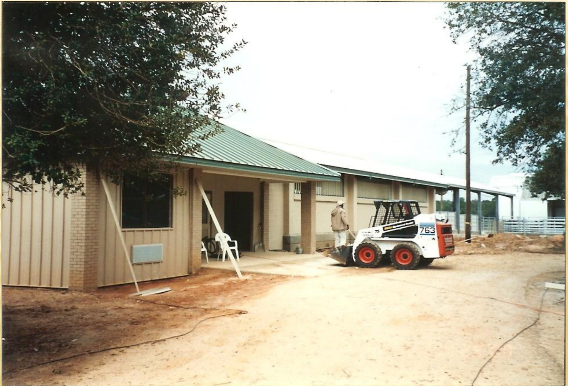
New Dairy Parlor Under Construction Franklinton, LA
